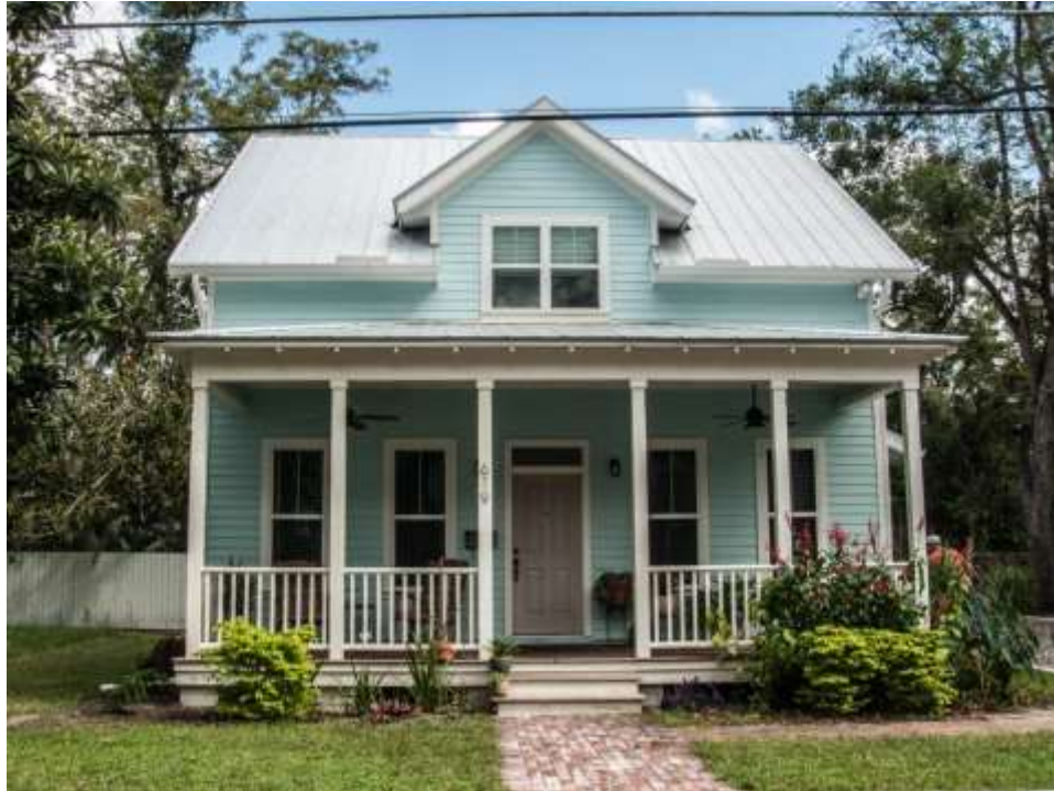
Fig. 5-15 619 NW 3rd Street (AL01490)
