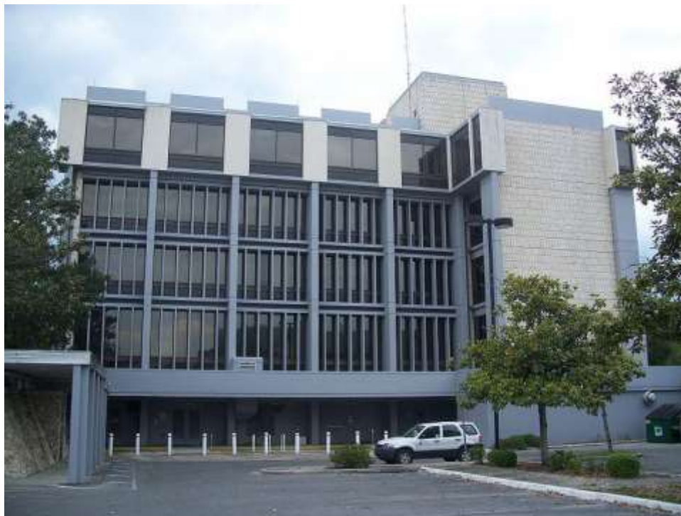
Fig. 5-1 Gainesville City Hall & Library (AL5855)
