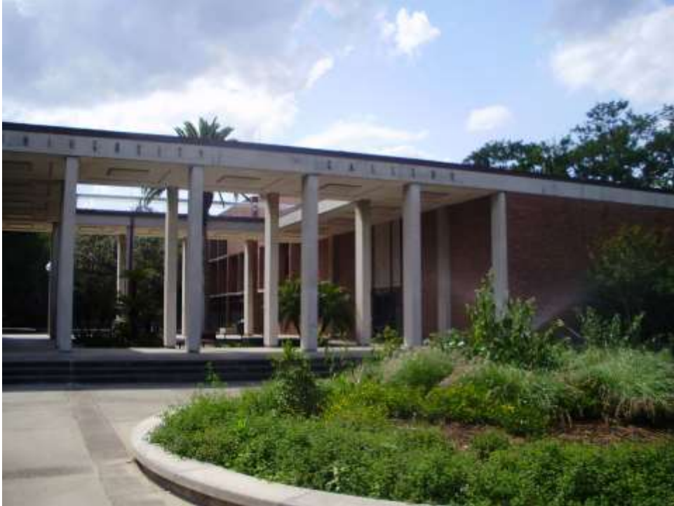
Fig. 5-2 UF Fine Arts Complex Building B (AL5858)
