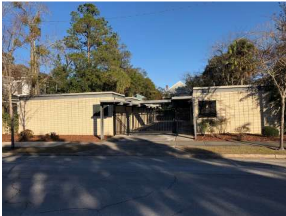
Fig. 5-20 519 NE 1 st Street (AL05904)
