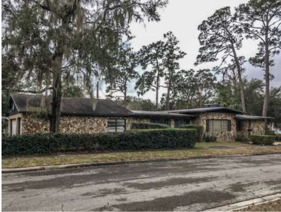
Fig. 5-16 537 NE 7th Avenue (AL03471)
