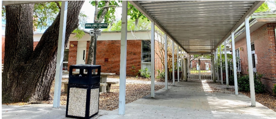
Figure 5-18 J.J. Finley Cafeteria Building 1949
