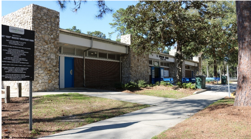
Figure 5-16 Westside Park Pool Building (AL07330)
